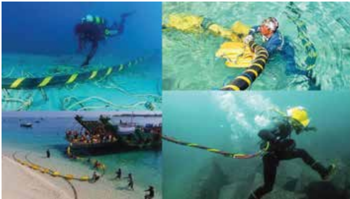
Figure 8 : Submarine Cables and Pipeline Laying (Symbolic Picture)
