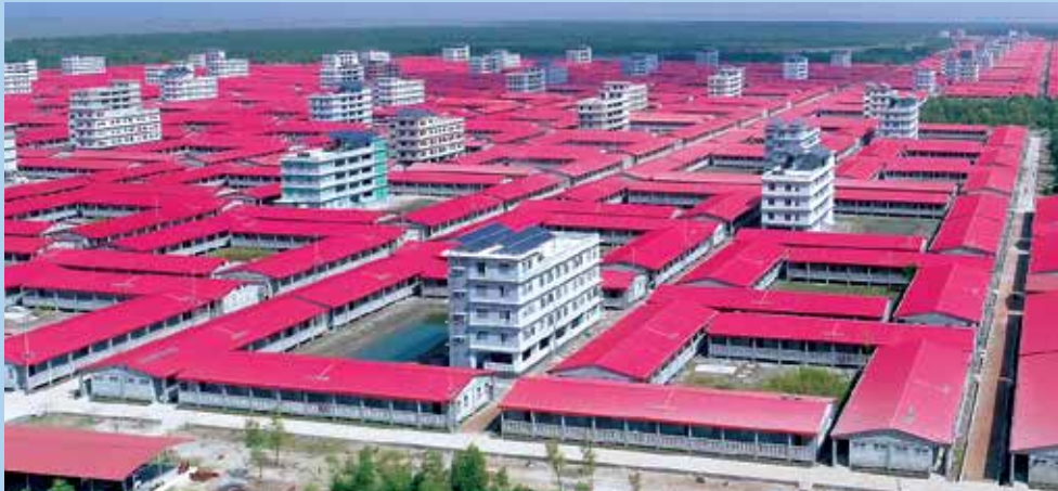
View of the cluster houses built on Bhasan Char
